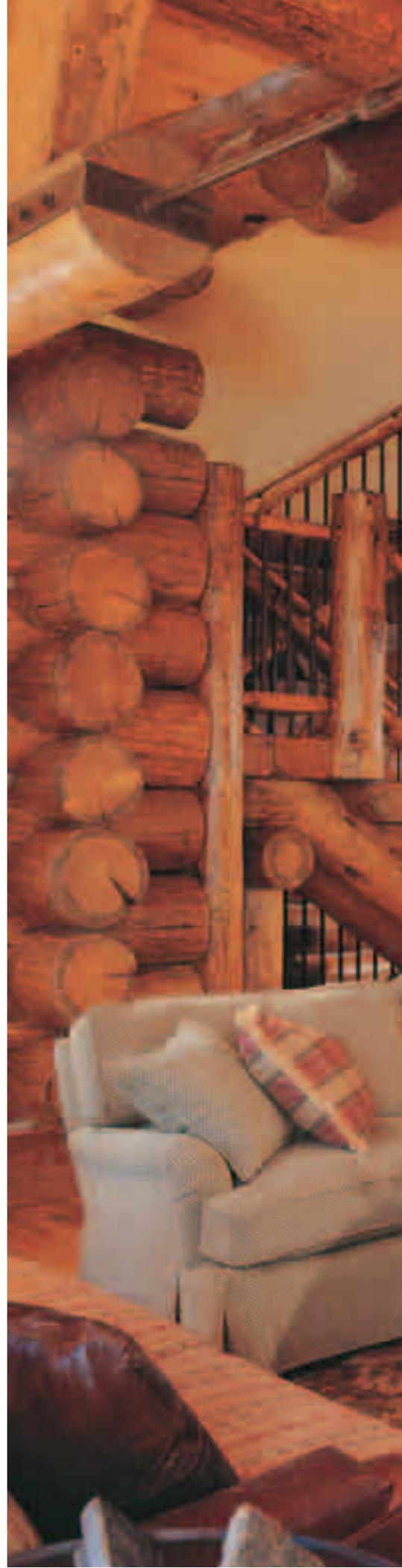
this handcrafted, chink-style home. Fourteen-inch diameter logs were used for the walls, while 18-inch diameter logs form the roof. “Even though the basic style includes chinking between the stacked logs, none of the column-to-beam work is chinked,” says Matt Lee, the owner of Teton Heritage Builders. “We crafted the log connections tightly so that fill was not necessary. This type of craftsmanship makes log-home construction an art form.”
