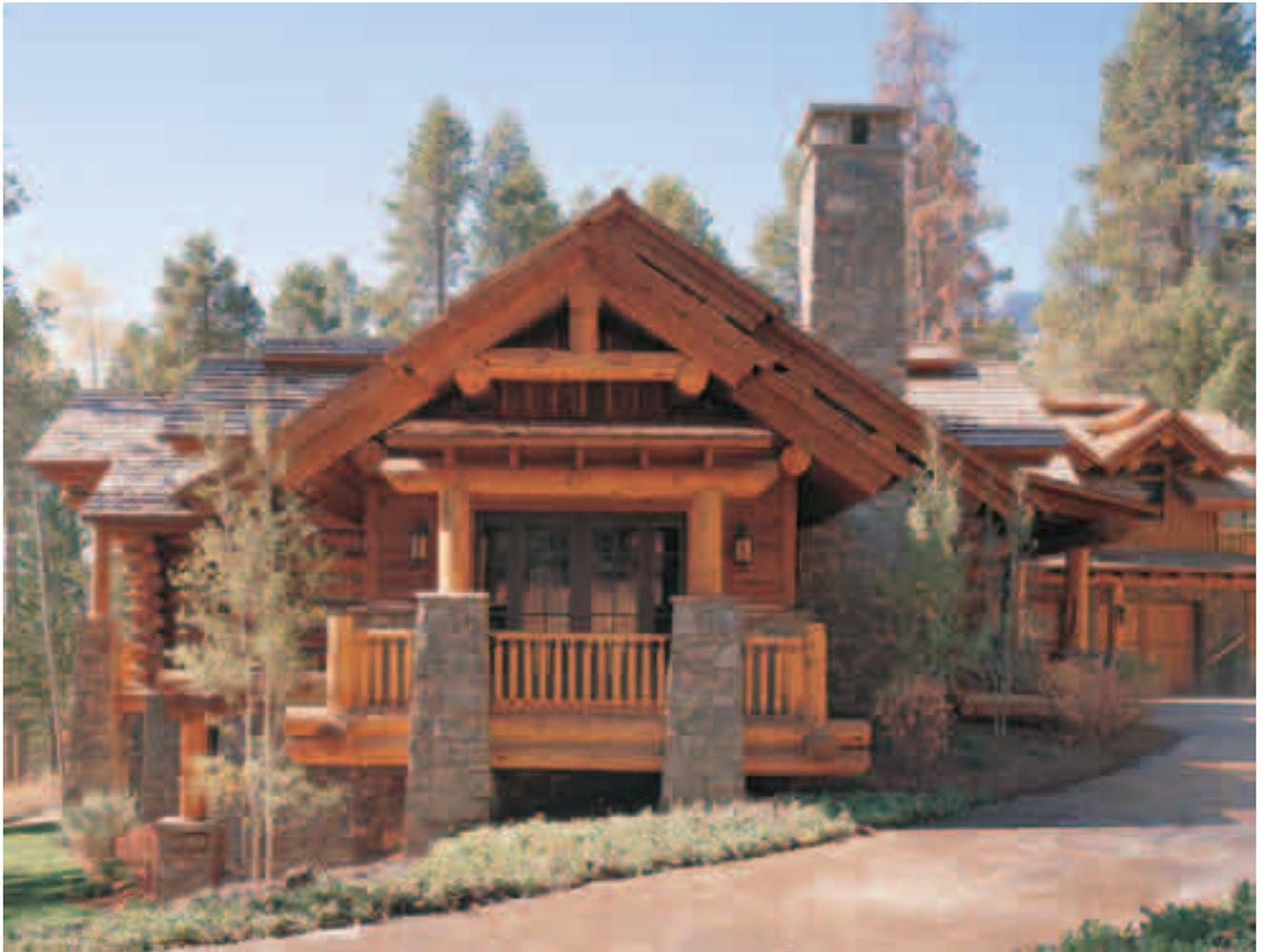
**The deck off the dining room features an exposed rafter shed-type roof supported by buttressed piers. Extending the structural ridgepoles and purlins creates a typical mountain cabin porch. Alaskan yellow cedar was chosen for all of the decks due to its durability when exposed to high-altitude sunlight.**
